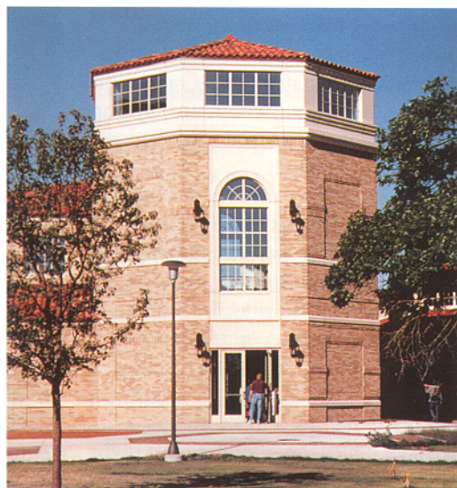
Ribbon-cutting for the Southwest Collection/Special Collections Building will occur in the spring. (Tech Photo)
